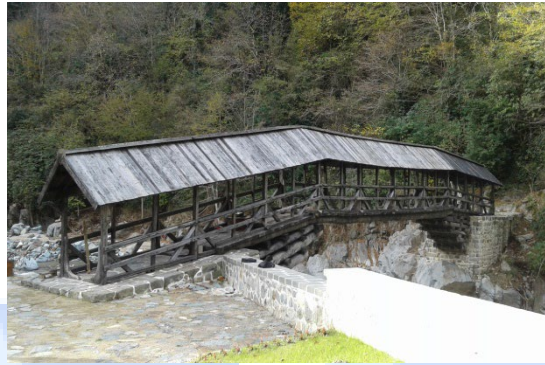
Figure 1. The Buzlupınar Bridge
