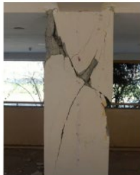
Classical failure of columns and shear walls due to several reasons: poor quality of concrete, columns does not having 135 degree hooks and having large spacing, etc.
