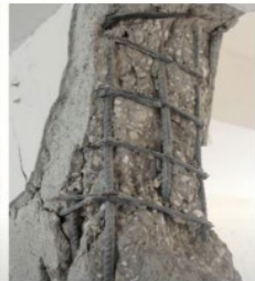
Classical failure of columns and shear walls due to several reasons: poor quality of concrete, columns does not having 135 degree hooks and having large spacing, etc.
