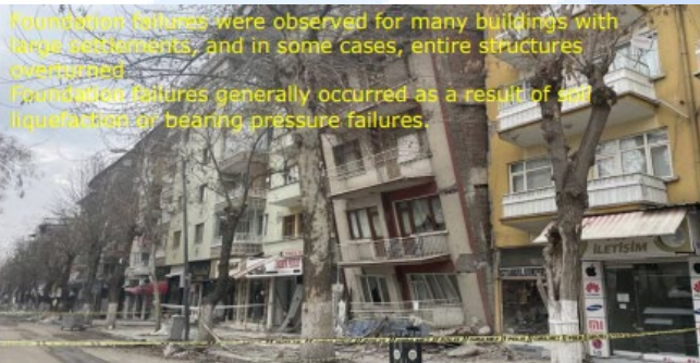
Liquefaction phenomena resulted in tilting of a building with no damage in the upper floors. Source: https://twitter.com/aysekarahassan/status/1623767921758461953
