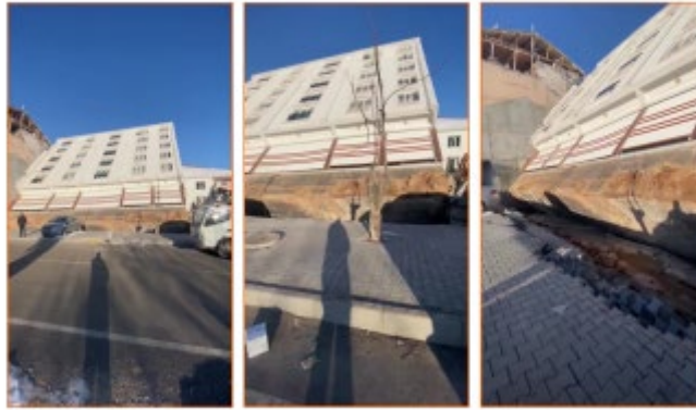
Liquefaction phenomena resulted in tilting of a building with no damage in the upper floors. Source: https://twitter.com/aysekarahassan/status/1623767921758461953
