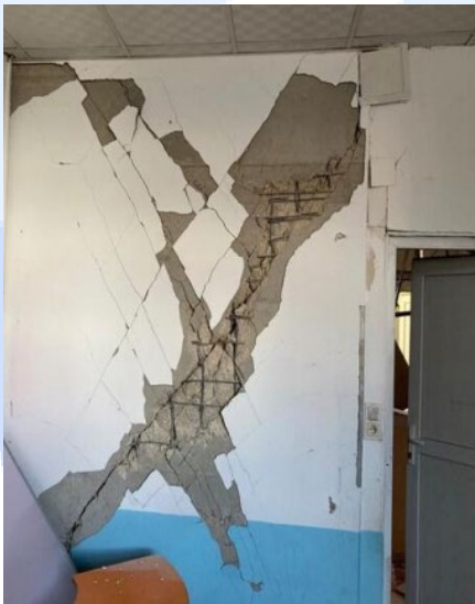
Lack of shear wall reinforcement anchorage
