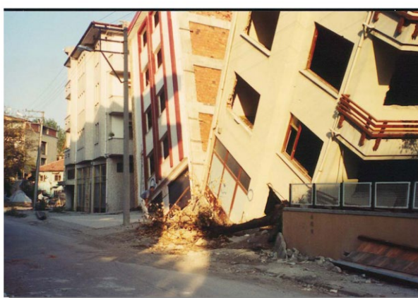
Figure 7. Liquefaction Damage, Adapazari, Turkey, 1999
