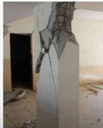
Classical failure of columns and shear walls due to several reasons: poor quality of concrete, columns does not having 135 degree hooks and having large spacing, etc.
