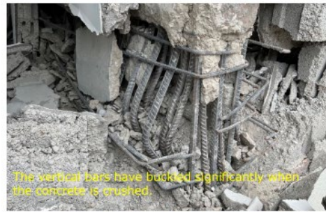
Typical deficiencies of the frame buildings constructed before 2000 were the use of plain reinforcing bars, insufficient steel reinforcement detailing and possibly low concrete strength resulting in heavy damage and collapse
