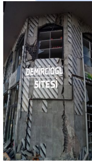
Lack of shear wall reinforcement anchorage
